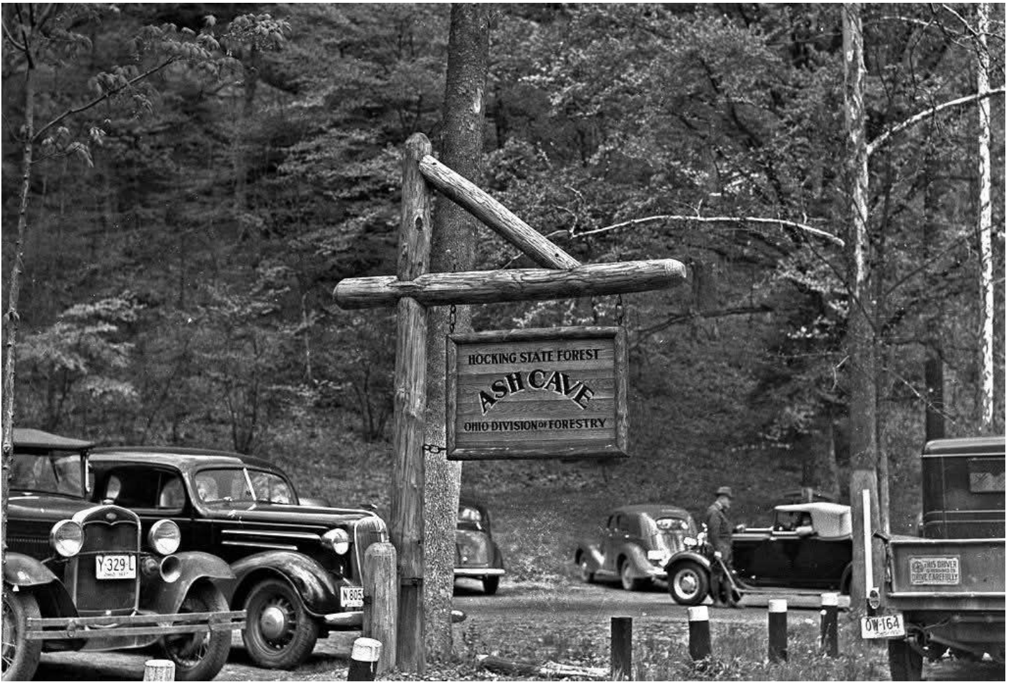
The parking area for Ash Cave in the Hocking Hills circa 1937. Columbus Navigator.
